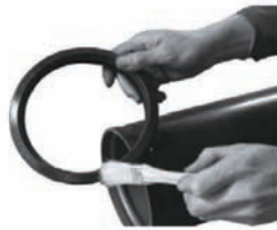
Lubricate gasket
